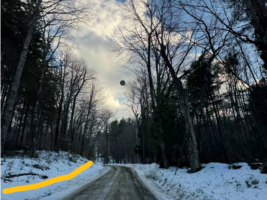
135501 before 1 - widen road 2-4ft and install stone line ditch on left side going uphill
