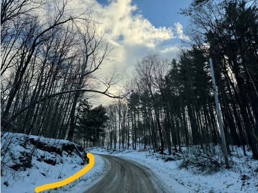
135500 before 2 - widen road 2-4ft and install stone line ditch on left side going uphill
