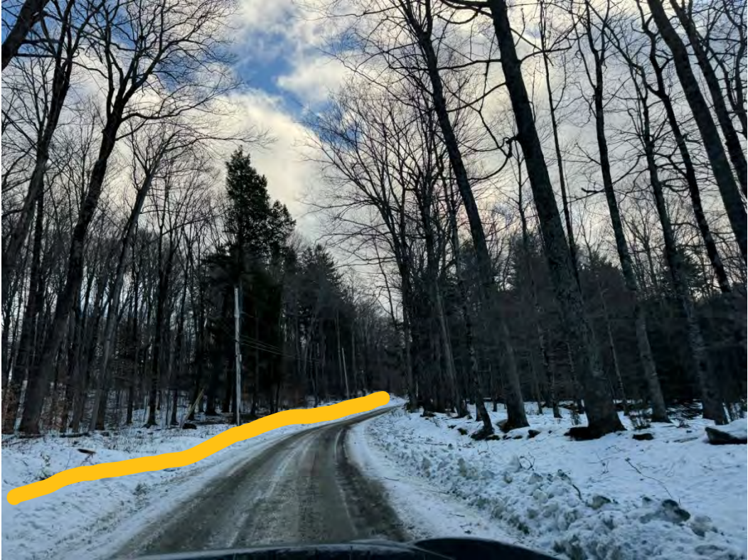
135502 before 2 - widen road 2-4ft and install stone line ditch on left side going uphill
