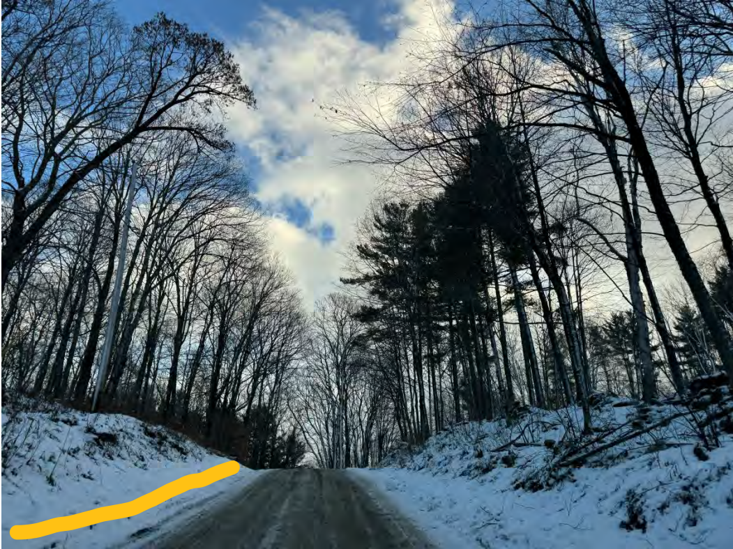
135499 before 1 - widen road 2-4ft and install stone line ditch on left side going uphill
